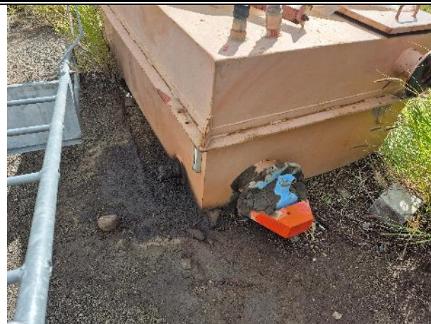
Oil tank spilling onto the soil
