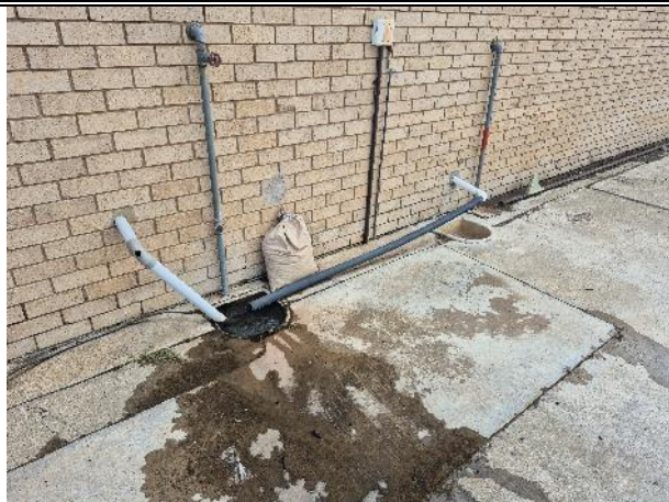
Blocked drain to be opened
