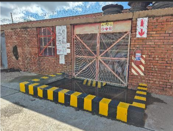
Wash bay drain to oil sump
